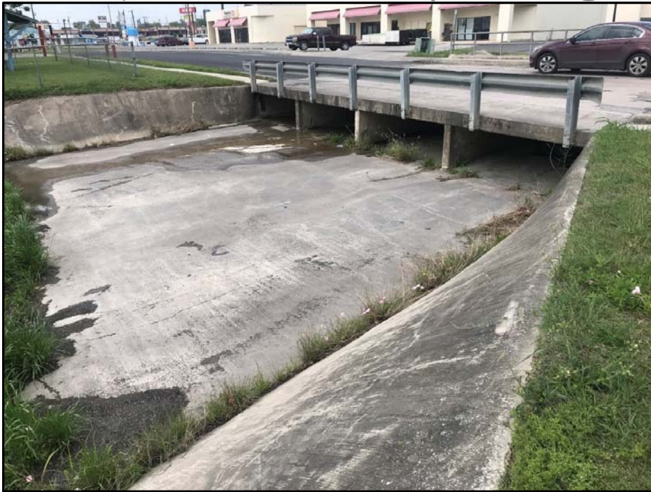
Existing Drainage Structure on Avenida Prima
